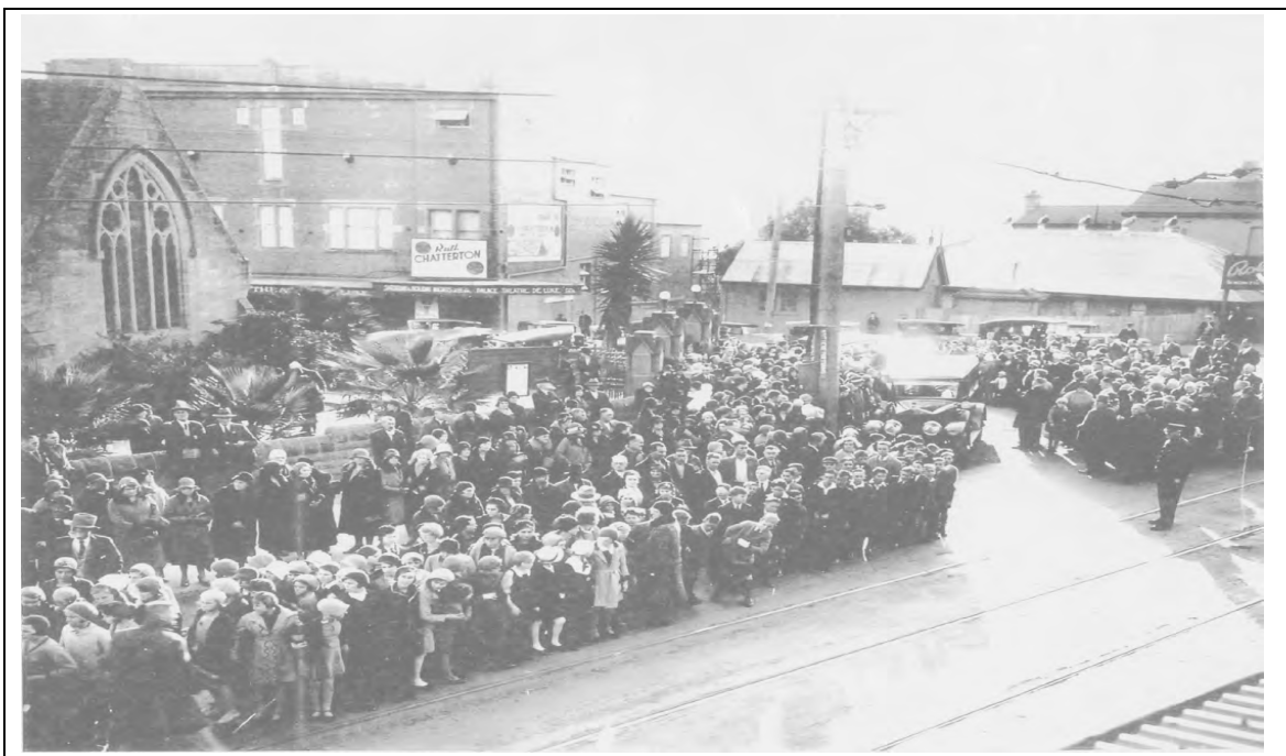
For decades the junction of Victoria Road and Jordan Street was characterised by the contrast between the antiquity of the sandstone Christ Church and modern, bulky façade of the now demolished Palace theatre at no. 1 Jordan Street. Other demolished structures of this by-gone era are the former tram waiting shelter and staff rooms and the Blaxland family's Karlite (no. 226-230 Victoria Road) shown at right of picture. Source: Ryde Library
