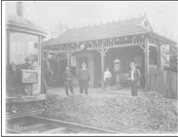
The Gladesville tram terminus at the corner of Jordan Street consisted of a weatherboard waiting shed, the starter and timekeeper's office, and staff toilet. Source: D. Keenan, The Ryde Line of the Sydney Tramway System , Sydney, 1988.
