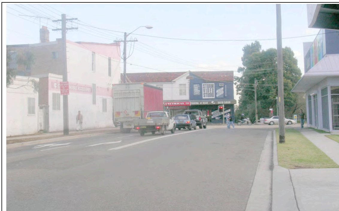
Monash Road looking south to the intersection with Victoria Road. The intersection is framed by buildings, two of which have historic value (no. 428-434 & no. 413-417 Victoria Road).
